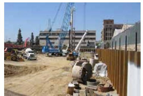
Excavation to P1 level
