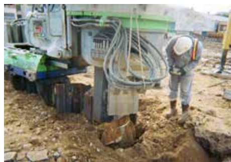
Installation of sheet piles
